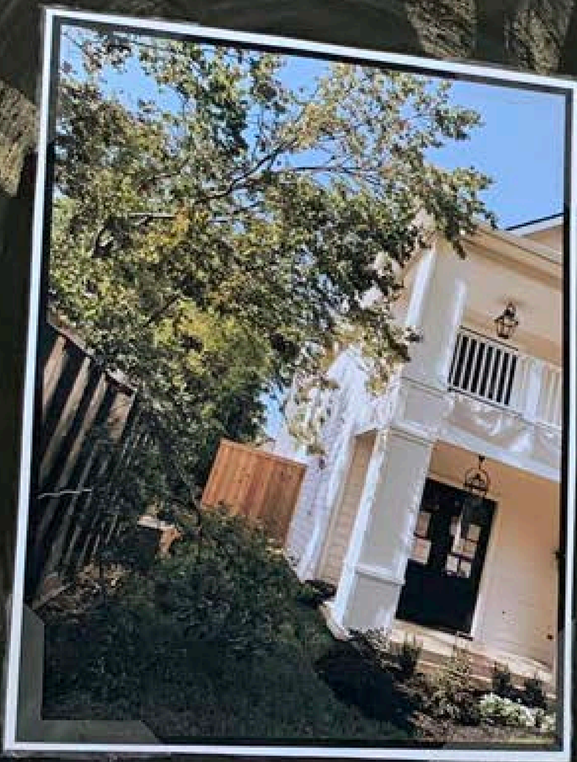
CUT TREE FELL ON NEW HOUSE
